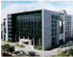
Taoyuan Technology Center (Green Building)
